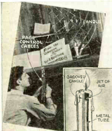
Above—How pages of a book are turned by flexible cables, the operator keeping out of camera range. Right—candle is extinguished by squeezing rubber bulb.
